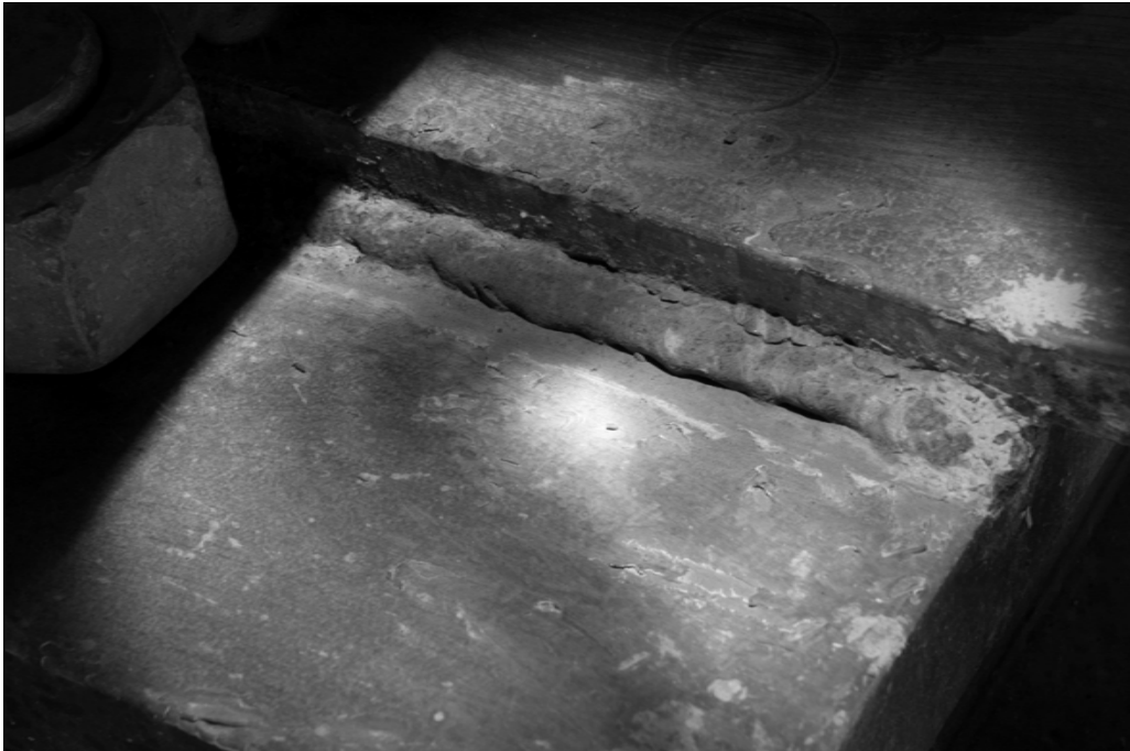
Unacceptable weld (overlap at the bottom toe, undercut at the top toe)
